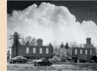
Above: Construction of the Willson Building at 230 North President Avenue. (1956)
